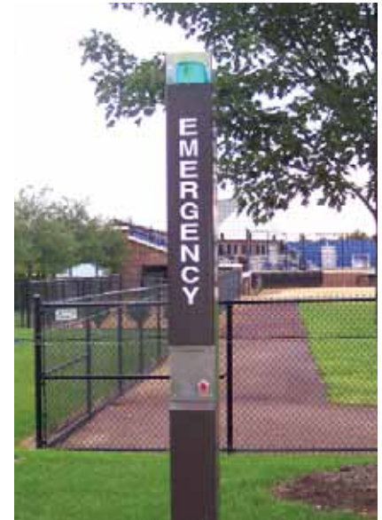
One of the many Blue Emergency Light Telephones on campus.
